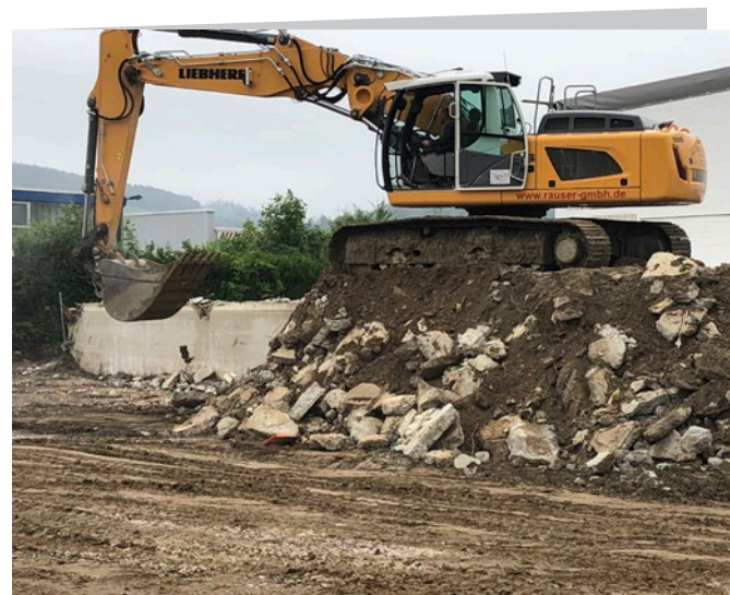
Deconstructions are carried out in a resource-friendly manner.
